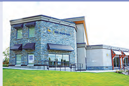
RBC at Roundabout Square 7188 West Saanich Road
